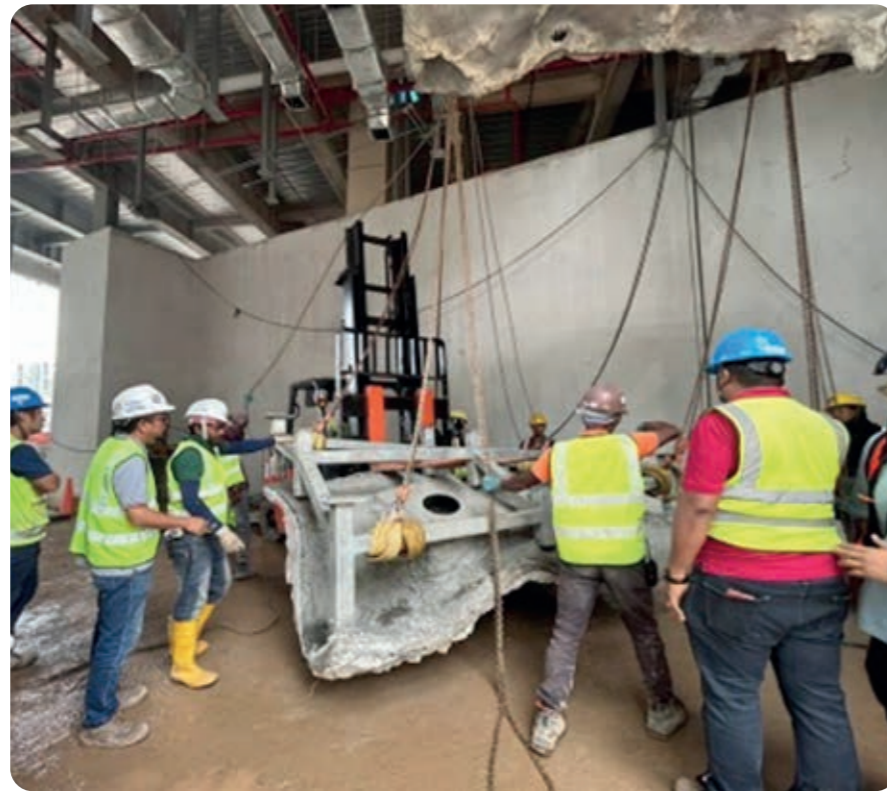
Installation of theming panels for the cavern at Rainforest Wild Asia
